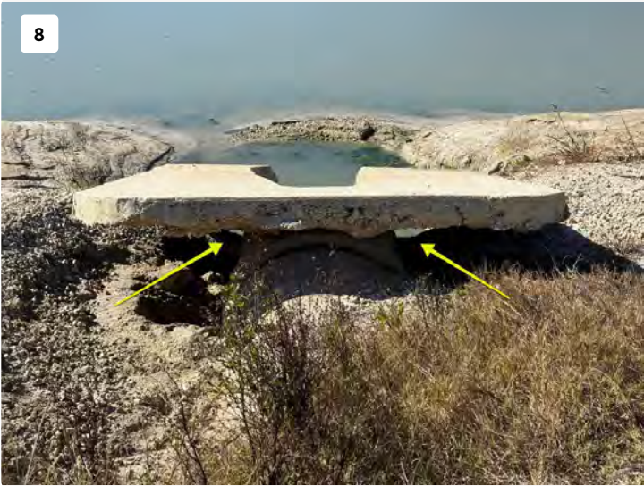
Water flow has scoured out the base material.
