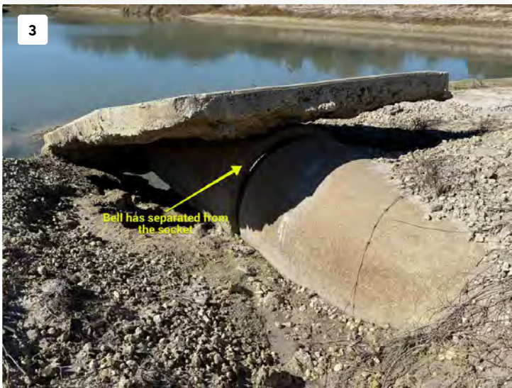
Inspection of the stormwater structure indicates failure of the concrete headwall/mitered end due to soil erosion and undermining. The mitered end has lost structural support and has partially separated from the main pipe (socket). Continued erosion is occurring around the pipe outlet, which could lead to further damage and complete collapse. The bell/socket on the main pipe is still good. This structure conveys stormwater runoff after rainfall events and is an important component of the community's drainage system. Recommend: We recommend removing the failed head...
